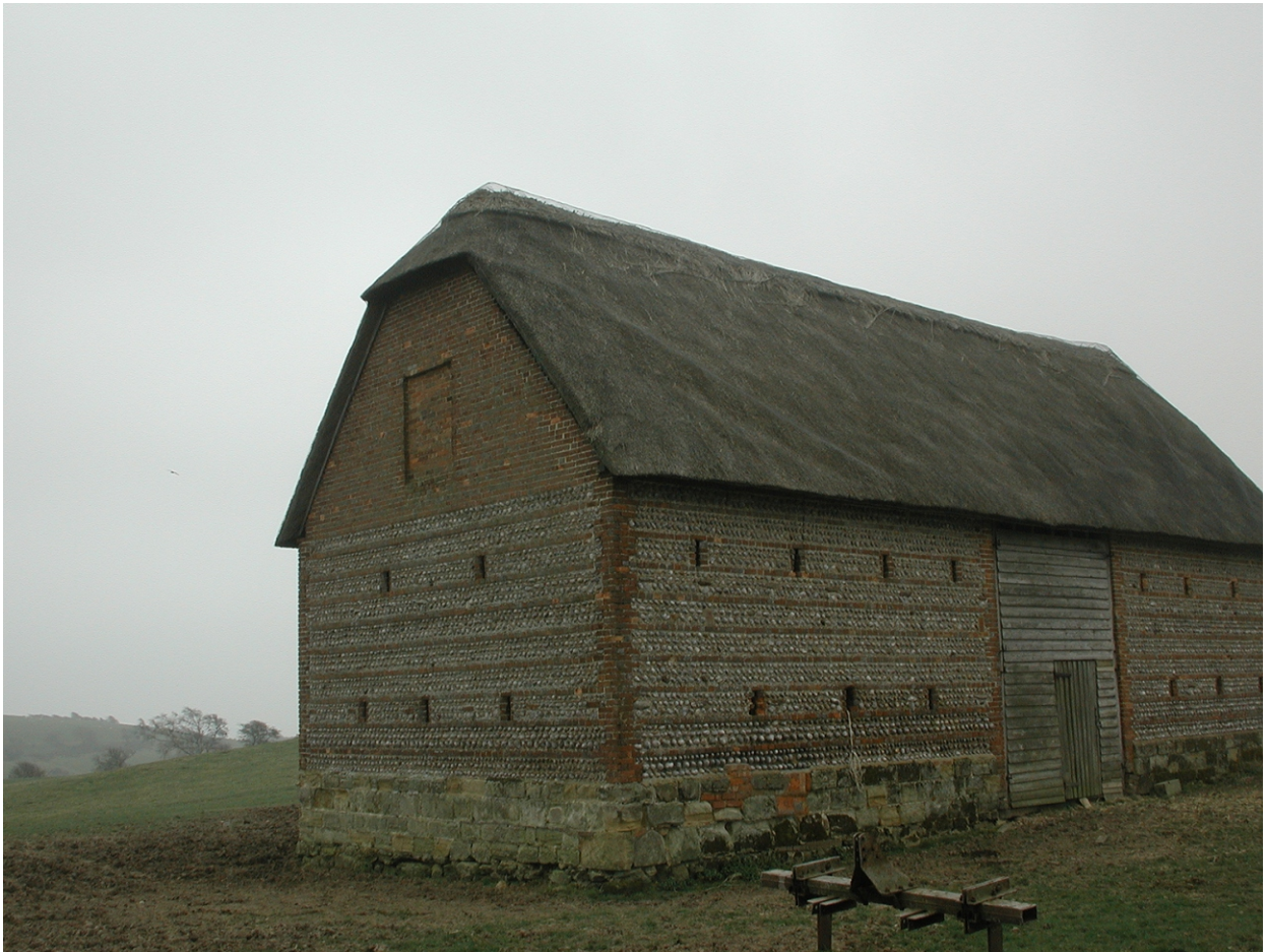
Plate 5. Old Marsham Barn detail of construction, north-western corner (NTSMR 129667).
