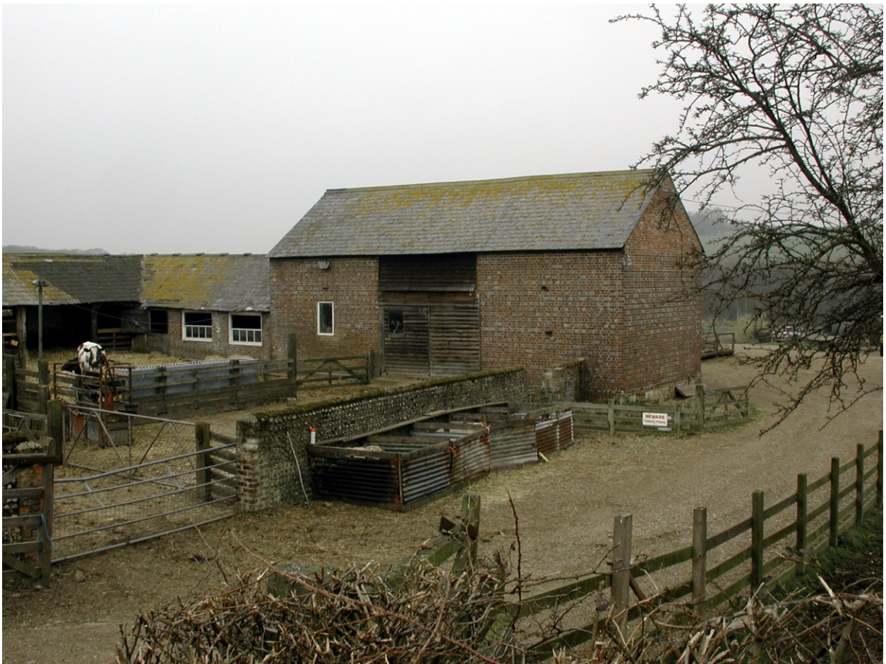
Plate 14. Old Marsham Farm, the Barn from the east (NTSMR 129674).
