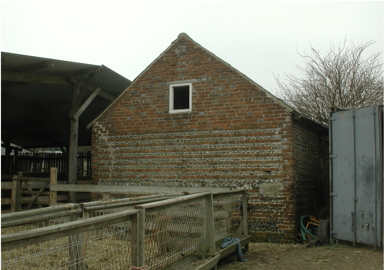
Plate 11. Old Marsham Farm, Sheephouse/calfhouse (NTSMR 129675) from the north-east, showing construction.
