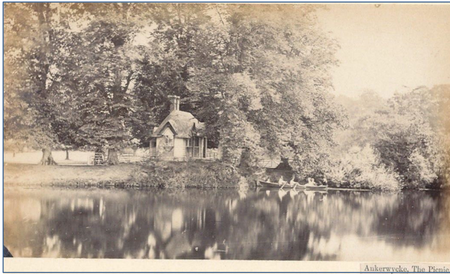
Figure 4.9. The Picnic House with the River Thames in the foreground
